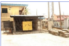
Uninterrupted Power Supply
